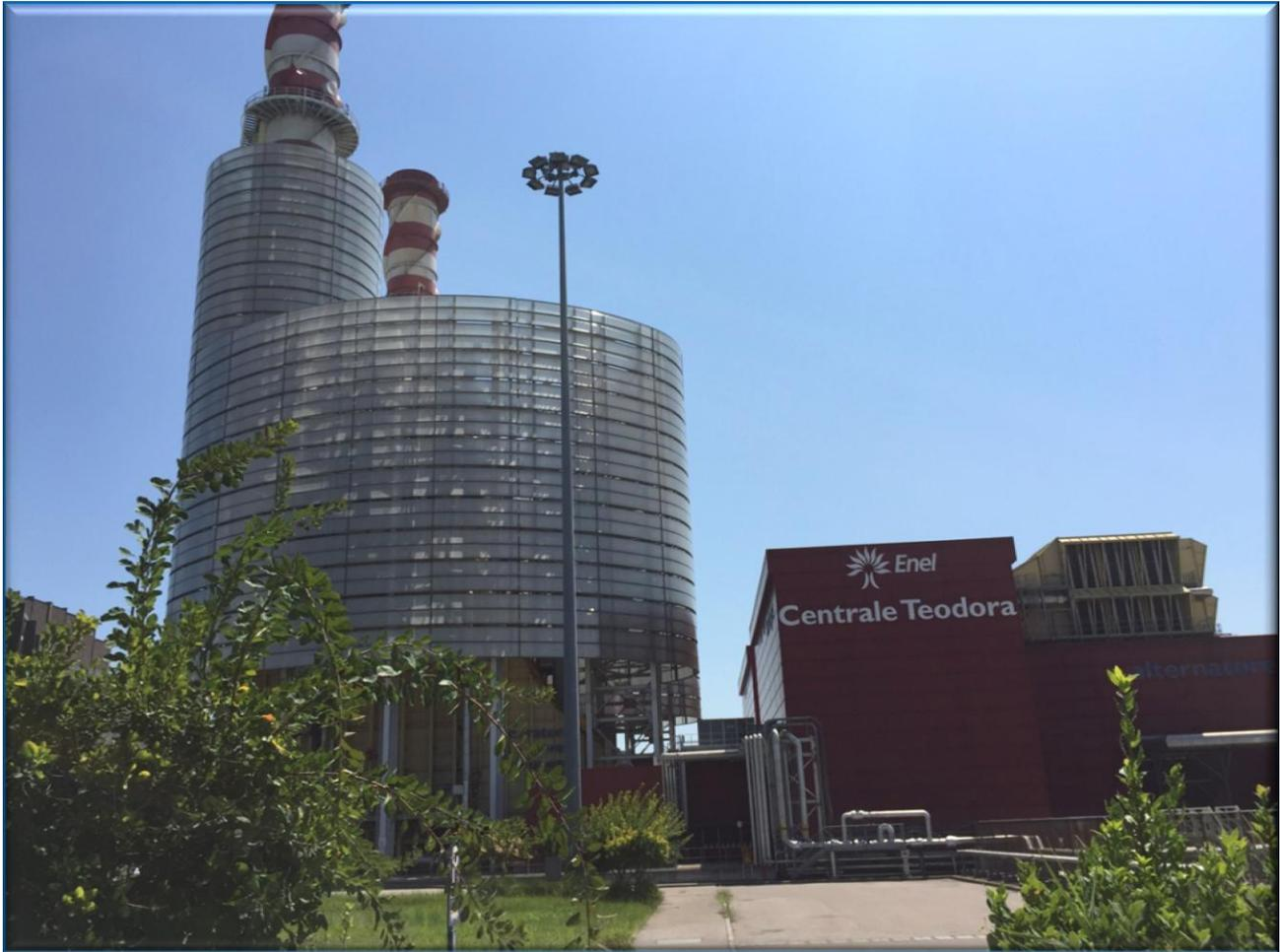
This is one of the most advanced power station of the big Italian Enel network; in fact the main Energy is produced by the first two Main gas-Turbines, while the steam, released by this first energy cycle, is conveyed to a second couple of Turbines in order to additionally produce electric energy with the recovered steam of the first cycle phase.
