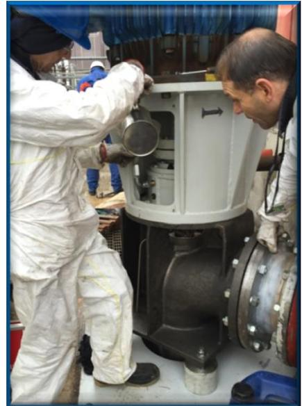
Here on the right is shown the pump installed, ready for the first start up hydraulic test.
